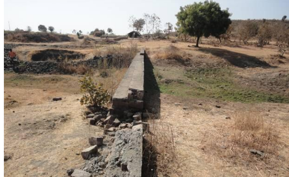
Damaged Check dam
